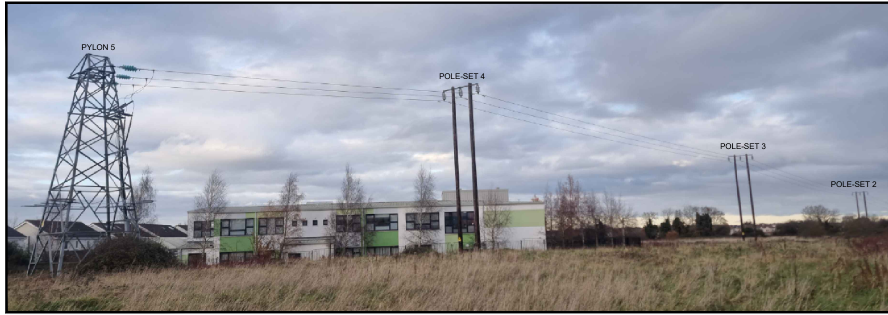
IMAGE OF EXISTING 38KV OVERHEAD SERVICES AT NORTH OF SITE TO BE UNDERGROUNDED
